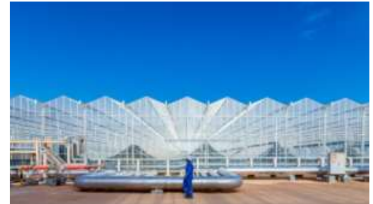
Miraah in Oman- the largest SHIP plant worldwide. Photo: Glaspoint
