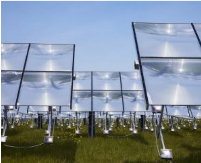
Concentrating collectors (Point Focus Fresnel) deliver heat at around 160 °C in Hørsholm, Denmark (Photo: Heliac)
