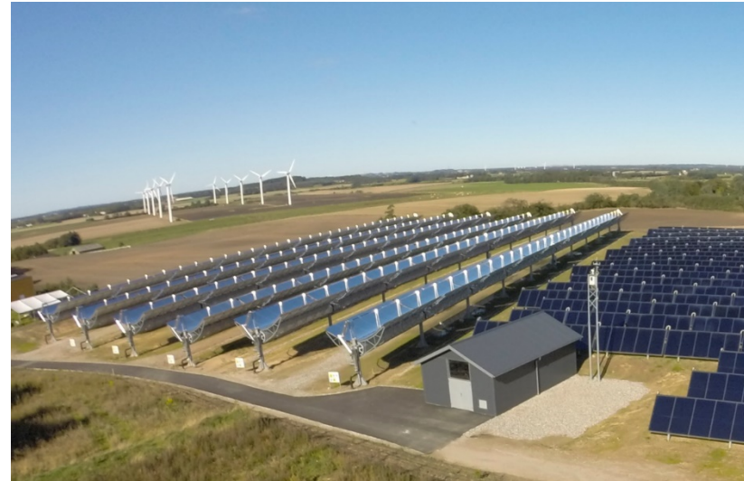
Combination of flat plate collectors (up to 70 °C) and parabolic trough collectors (operated at 95 °C) in Taars, Denmark (Photo: Aalborg CSP)
